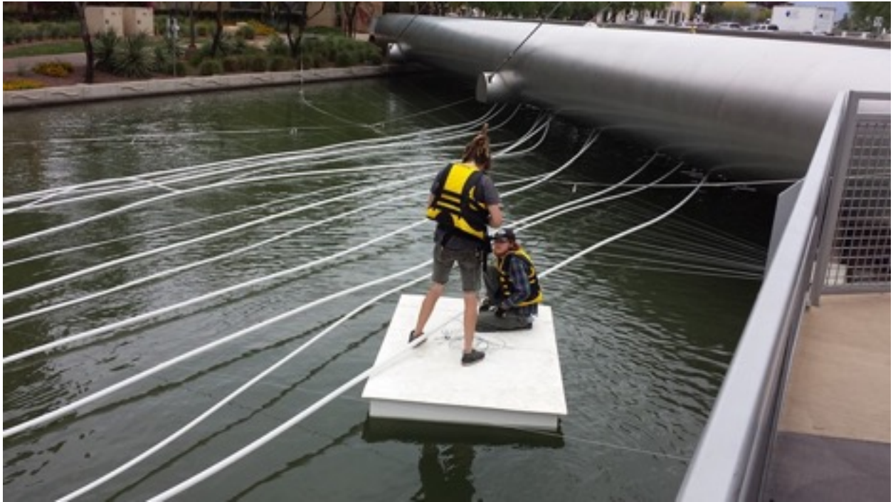
The installation team uses a pontoon to access various elements of the Golden Waters sculpture.
